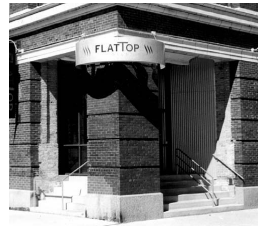
New Business Signage
